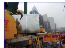
Engine Noise Enclosure
