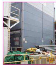
Construction Noise Enclosure
